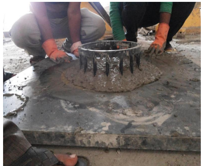
Fig. 3. Abrams Slump Flow Equipment.
