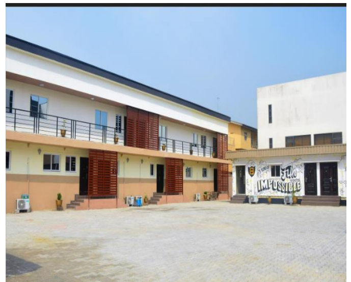
Fig. 3.3 Tempohousing Nigeria source: https://www.livinspace.net/
