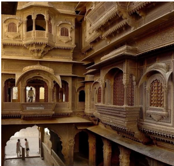
Figure 2. The sandstone facade of Patwon Ki Haveli, Jaisalmer (c. 1805). The 600–900 mm thick sandstone walls create a 10–12 hour thermal lag, while intricately carved jali screens admit diffused light and enable cross-ventilation.
