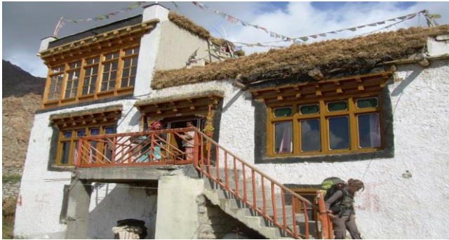
Figure 4. A traditional Ladakhi dwelling at altitude above 3,500 m. Thick mud-brick walls (500 mm), south-facing orientation, and small north windows form a passive solar heating system achieving indoor temperatures of 15–18°C in -20°C winters.
