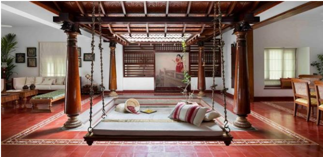
Figure 1. Traditional Nalukettu courtyard house in Kerala showing the central nadumuttam, steeply pitched clay-tiled roof, and timber columns. The open courtyard drives natural ventilation, maintaining indoor temperatures 3–5°C below ambient in peak summer.
