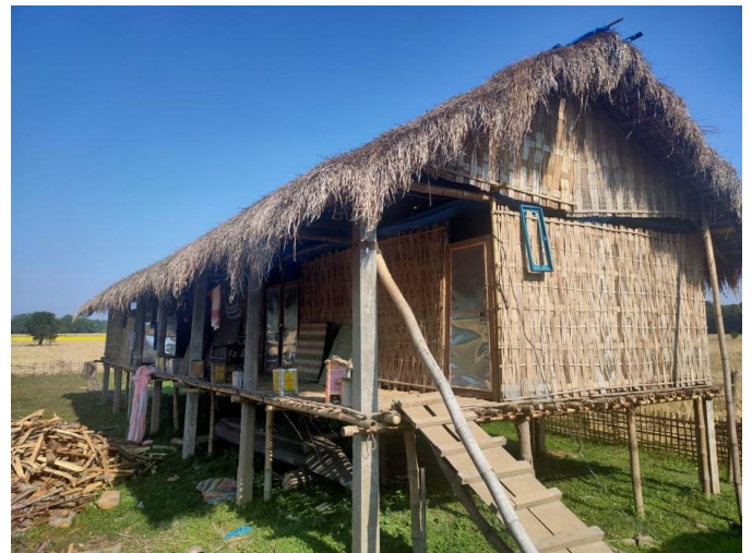
Figure 3. A traditional Chang Ghar stilt house in Assam, constructed from bamboo. The elevated platform protects against annual flooding, while bamboo's tensile strength (approximately 370 MPa) provides earthquake resilience. Open wall panels enable cross-ventilation.
