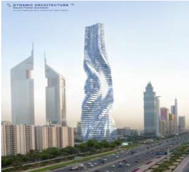
Figure 1. Conceptual rendering of the Dubai Rotating Tower, showing the dynamic, continuously changing form achieved by independently rotating floors around a central core.
