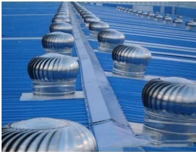
Fig 2 Roof Ventilators
