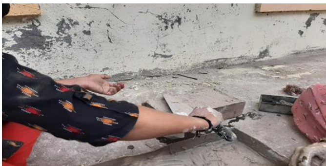
Figure22: Filling the mixture in the mould
