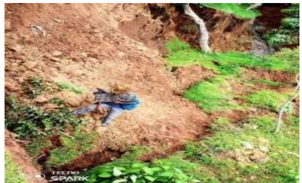
Figure 1: Surface damage due to landslide of Fudale landslide
