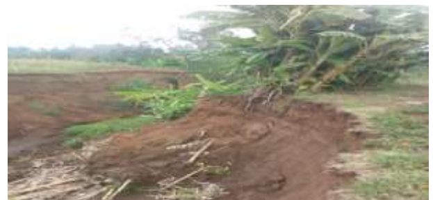
Figure 2: Destruction of plants and fruits due to landslide of Fudale Landslide
