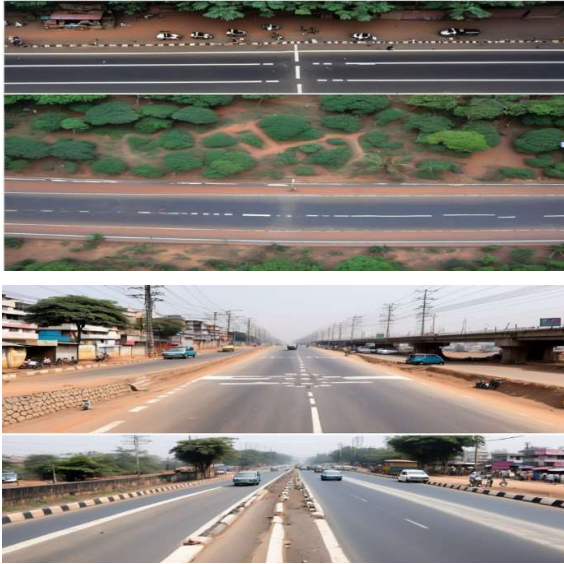
Figures: 3 Photos showing critical sections of road infrastructure.
