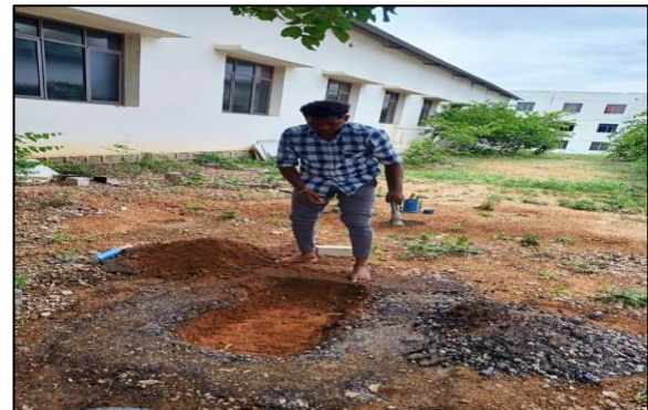
Fig.7 Base course Removal
