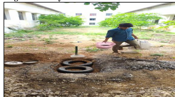
Fig.8- Placing used tyres.
