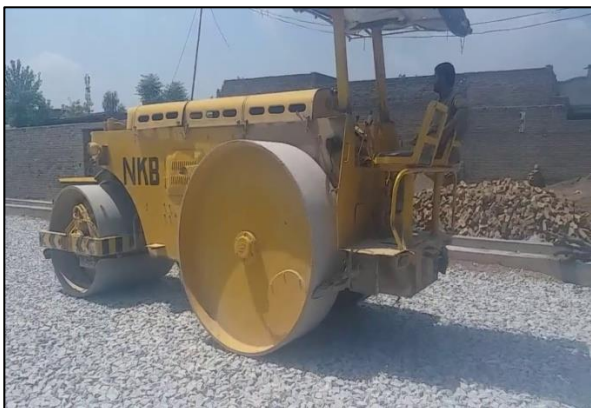
Fig.10 Compaction of Base course
