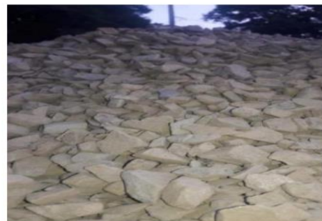
Fig.1 Concrete boulders obtained from demolished structures.
