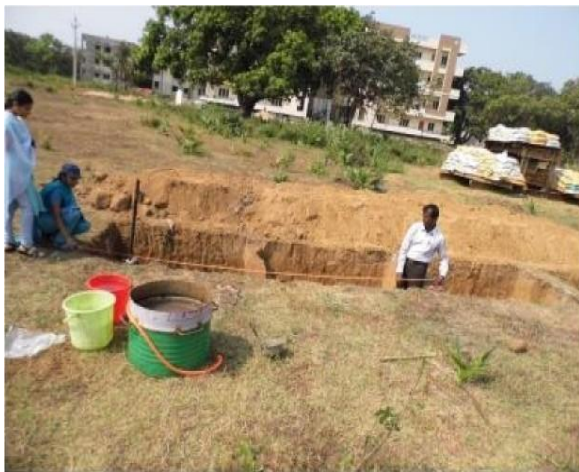
Fig 5. Plate 4.2 Open cut for field test track.
