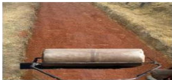
Fig 9. Plate 4.7 Subbase compaction with hand roller.
