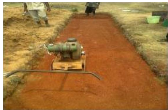
Fig 8. Plate 4.6 Subbase compaction with earth rammer.
