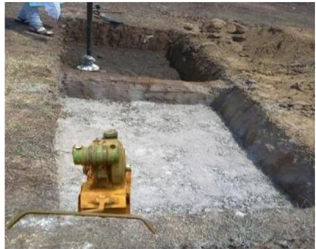
Fig 7. Plate 4.5 Flyash mixing with expansive soil.
