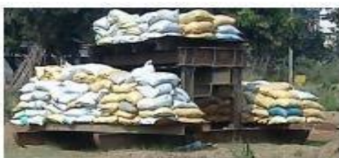
Plate 4.11 Loading Platform with sand bags
