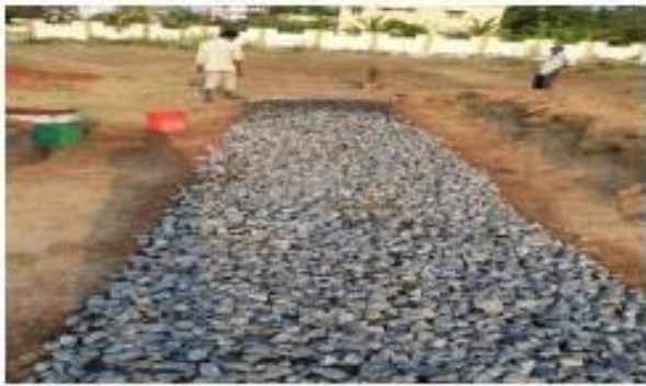
Plate 4.8 Process of laying the Base Course
