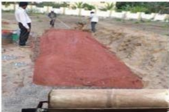
Plate 4.9 Completed Field Test Track
