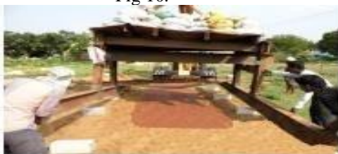
Plate 4.10 Installation of loading platform on Field Test Track
