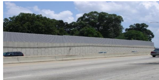
Fig.1. Highway sound barriers.
