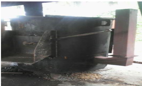
Fig 7. Plate 5: Boiler/Sterilizer (Source: Field Survey 2016)
