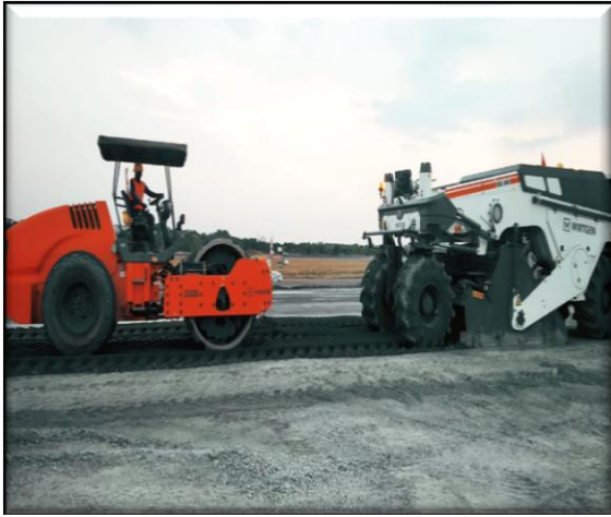
Fig .2. Construction of Asphalt Pavement - Gmr, Rgia Hyderabad
