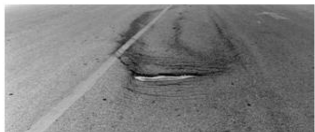
Figure 1. Slippage Crack.
