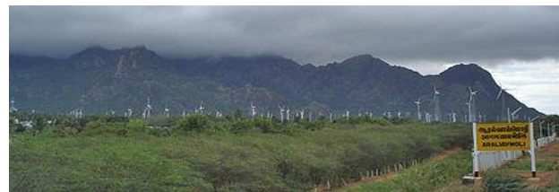
Fig.7 The largest wind farm of india in Muppandal ,Tamil Nadu.
