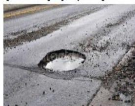
Fig.2. Pothole due to poor quality of material
