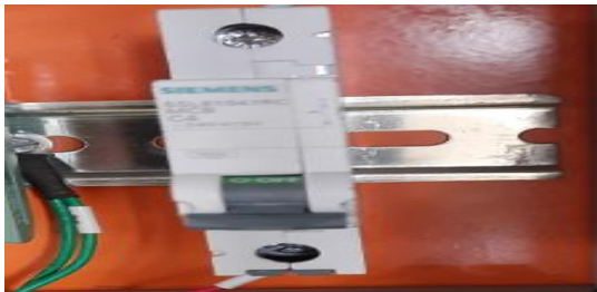
Fig.3. Miniature circuit breaker.
