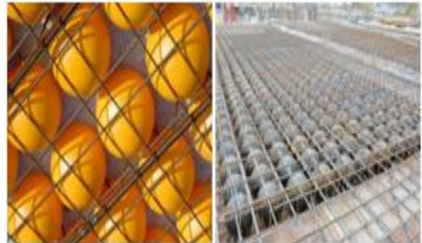
Fig.1 Bubble Deck Slab.
