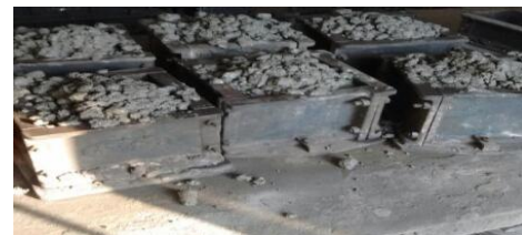
Fig.7 Vibration of Concrete
