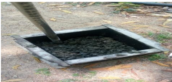
Fig.2 Compaction Of Concrete
