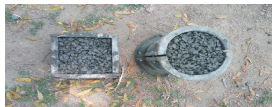
Fig.3 casting of concrete.
