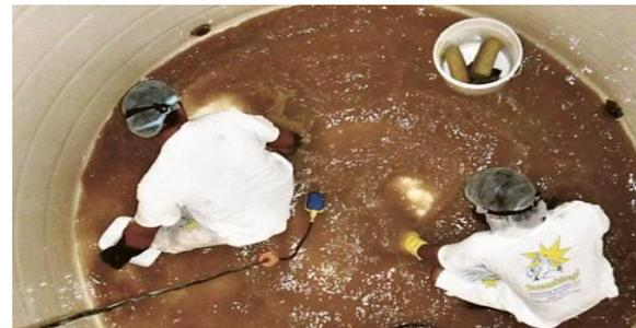
Fig.1 Manual Cleaning of water tank
